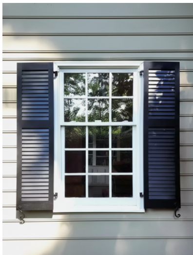
Shutter pairs from 12" - 48" in height require the use of 2 pairs of hinges/pintles
